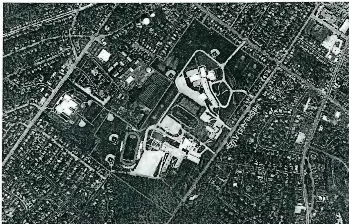
Abington High School Building Additions 170271001
