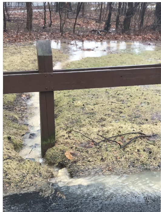
Photos: (left) Parking lot is pitched towards Forrest Ave. (right) Drainage is conveyed through an eroded channel.
