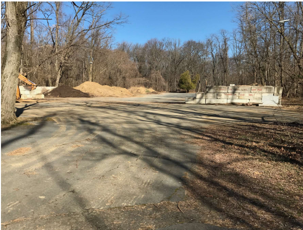
Photo: Parking lot and stockpile storage areas are included in the contributing drainage area to the rain garden.
