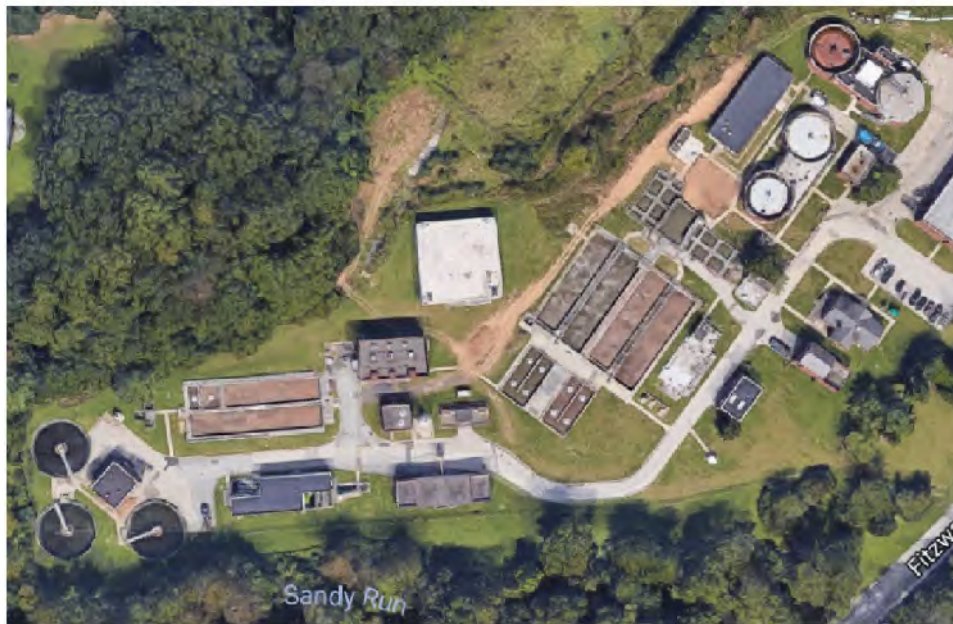
Figure A3-7: Abington WWTP including detailed schematic of the treatment process (top) and map of the site (bottom; map downloaded from maps.google.com)
