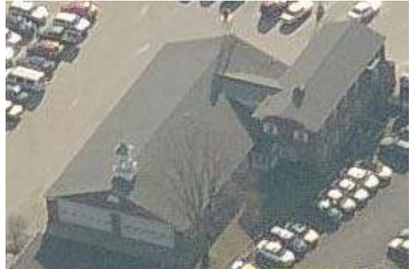
Figure 2 Station 100 Abington Fire Company
