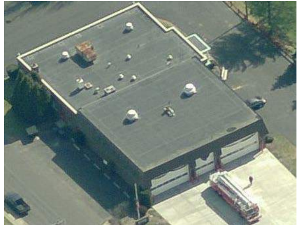
Figure 3 Station 200 McKinley Fire Company
