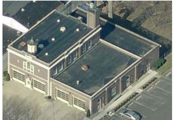
Figure 4 Station 300 Weldon Fire Company
