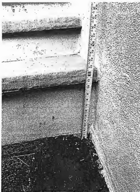
Figure 1: Front Porch Stair Measurement, 1st Step from Ground.
