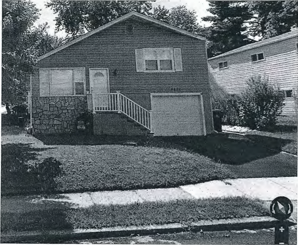
Figure 4: 2822 Jefferson Ave Pre-existing Porch
