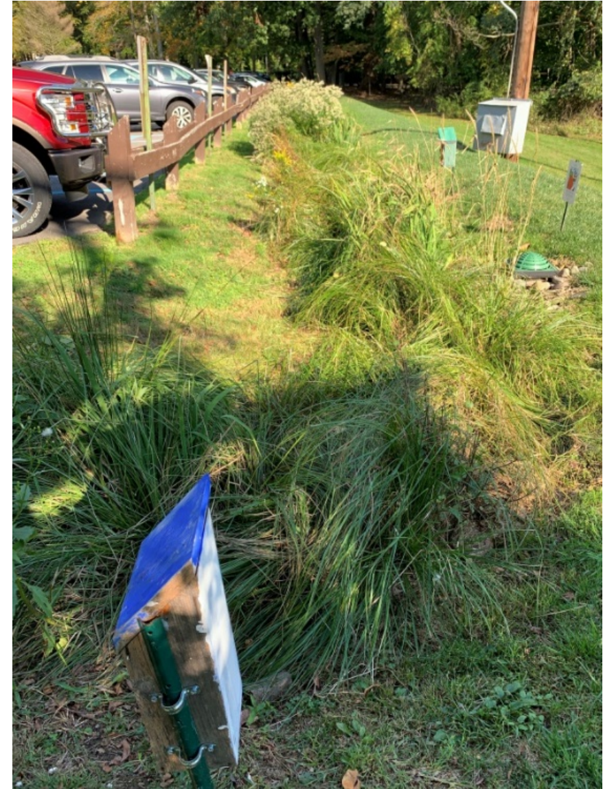
One Example of Environmental Sustainability Measures is the Bioswale Along the Parking Lot at Alverthorpe Park
