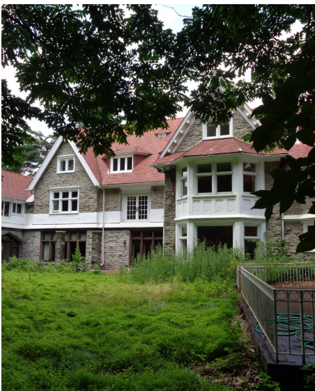
This residential structure at Susquehanna and Rydal Roads was demolished. A historic preservation ordinance could incentivize preservation and reuse of such structures.
