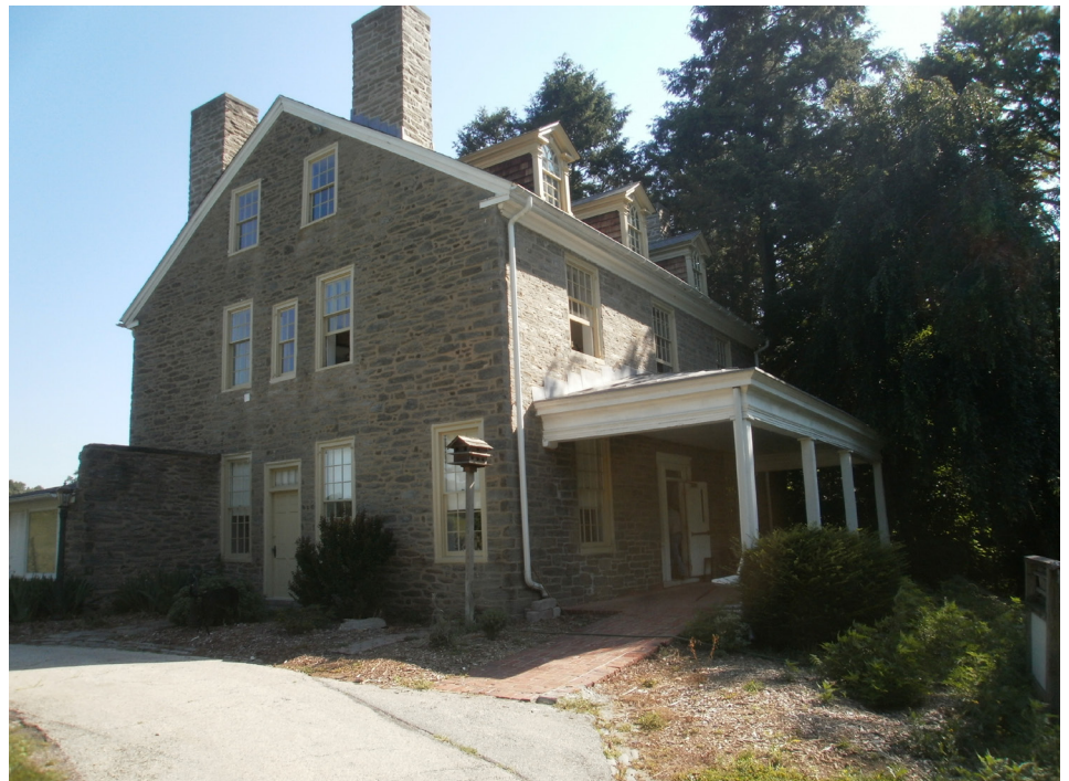
Fox Chase Farm manor house, 8500 Pine Road (listed on National Register)
