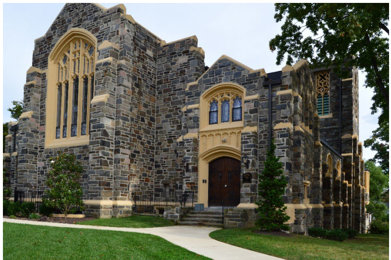
Narberth Place is an example of adaptive reuse. This reuse project converted a vacant church and rectory into residential units in Narberth Borough.
