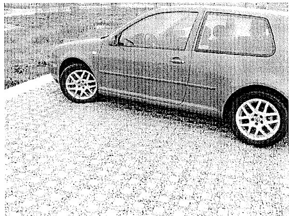
Example of a parking lot made with geo-pavers.
