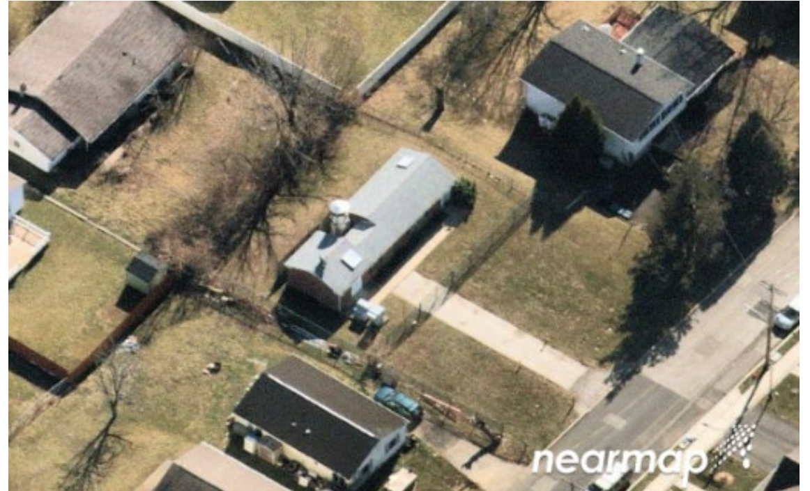
The North Hills Well is Being Upgraded for Advanced Filtration
