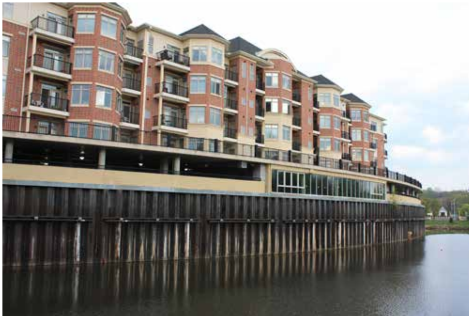
Figure 14.2 Elevated Structure, Pennypack Creek
