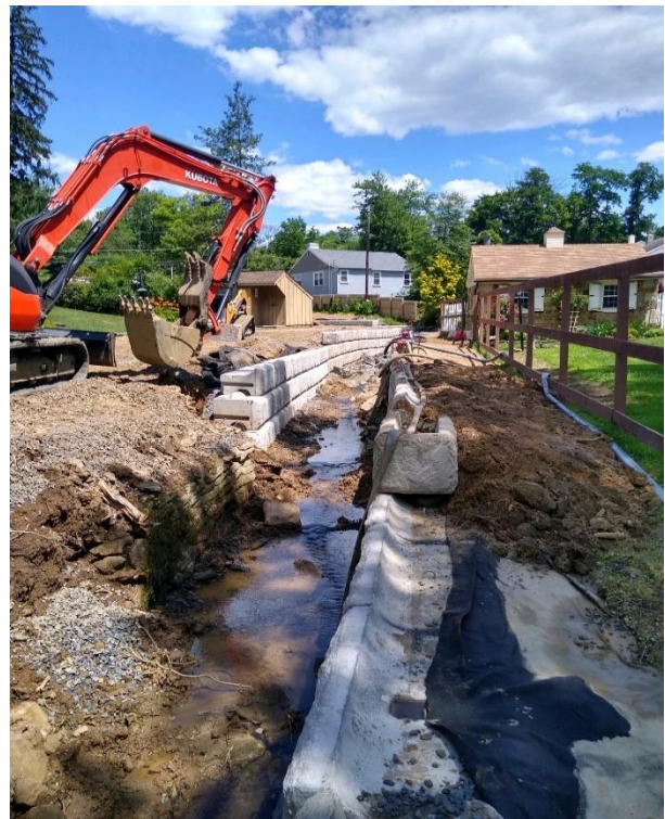
Old Huntingdon Pike Streambank Stabilization Project.
