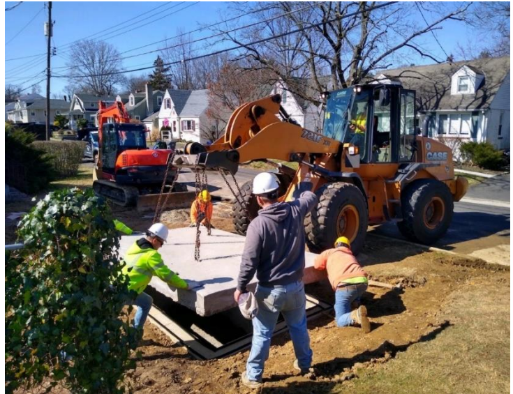
Hamel Avenue storm sewer project.
