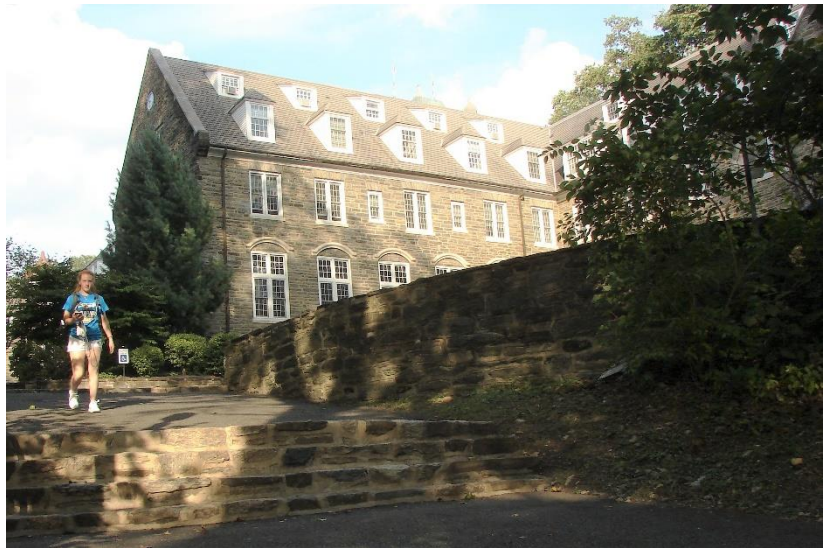
Sutherland Building, Penn State-Abington
