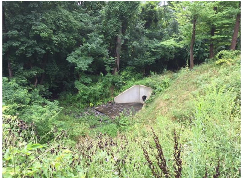
Stormwater Outfall Behind Lion's Gate Apartments
