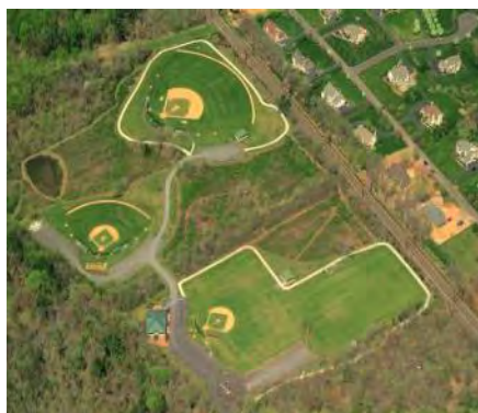
The SC plan for Penllyn Woods Park placed 4 play fields on uplands within a 75 acre site composed mostly of wetlands.
