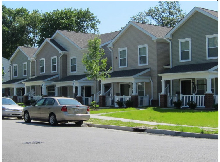
Crest Manor was designed to obtain LEED (Leadership in Energy and Environmental Design) certification
