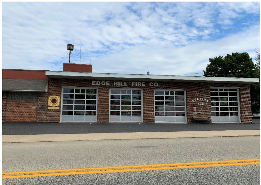
Edge Hill Fire Department, North Hills.
