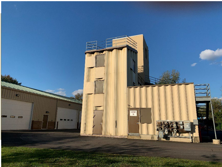
The Township's Fire Training Facility, Florey Road
