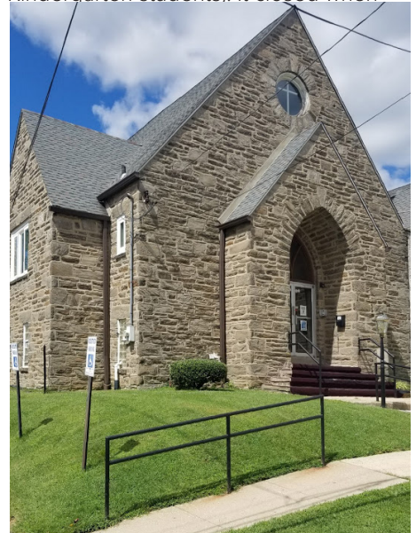
The First Baptist Church of Crestmont was constructed 1910-1919 to serve the African-American community between.
