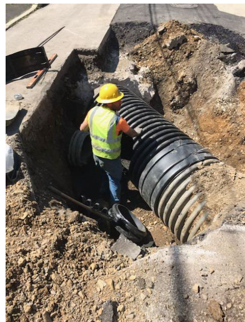
Figure 6-2: Hamel and Monroe Avenue Flood Control Project
