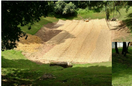
Figure 2-6: Melmar Basin: Grade, repair, and stabilization improving flow management and water quality discharge
