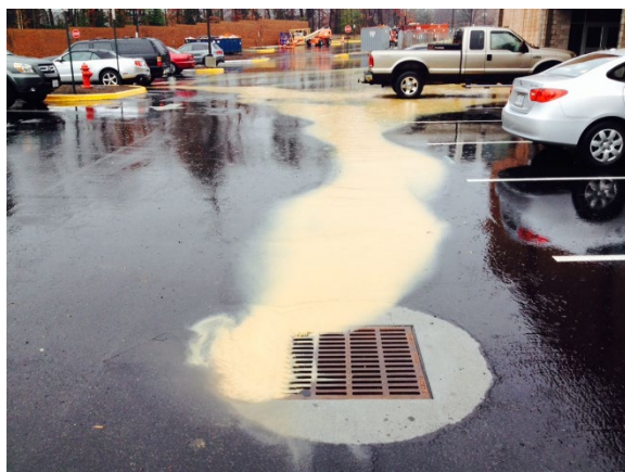
Figure 2-4: Sediment runoff from a nearby construction site to a stormwater inlet structure.
