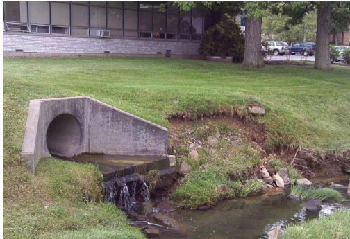
Figure 2-1: Stormwater inlet/outlet structures.
