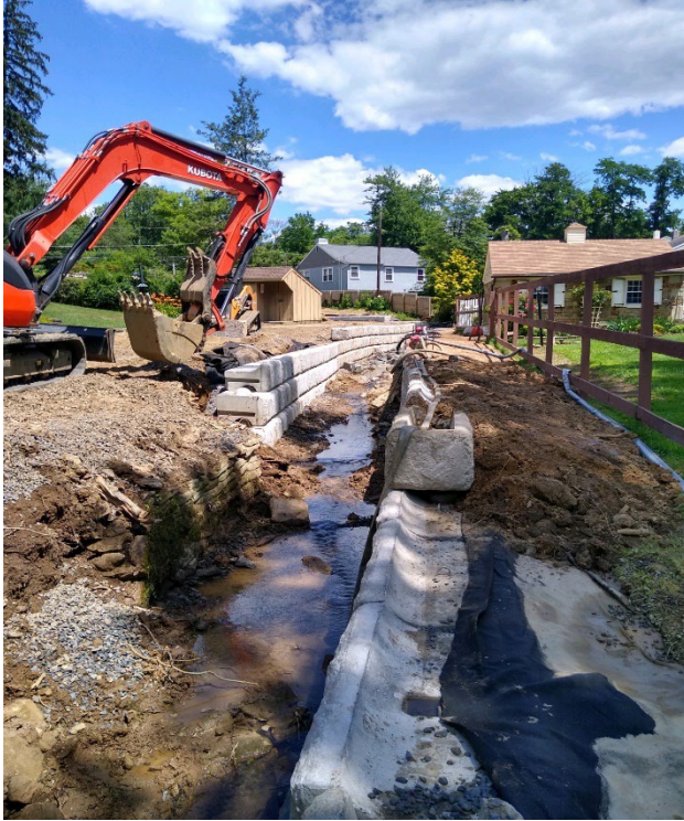
Figure 6-3: Old Huntingdon Pike Stream Bank Stabilization
