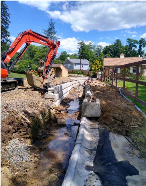
Figure 2-2: Old Huntingdon Pike Stream Bank Stabilization
