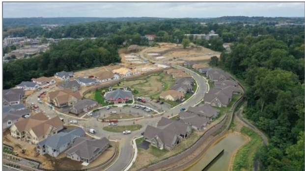
Rydal Waters, a senior living cottage development, opened in 2020 in the northern part of the study area
