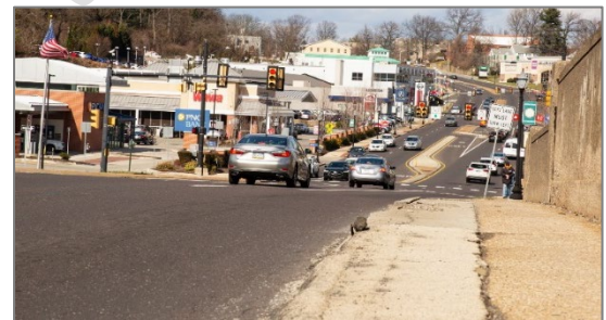
Poor sidewalk conditions
