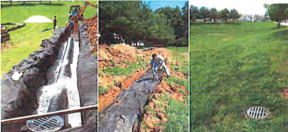
Figure 3: Example of Infiltration Trench Installation
