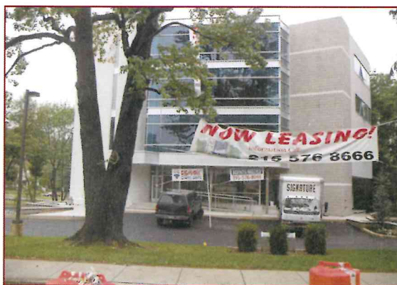
New office building at 1021 Old York Road
