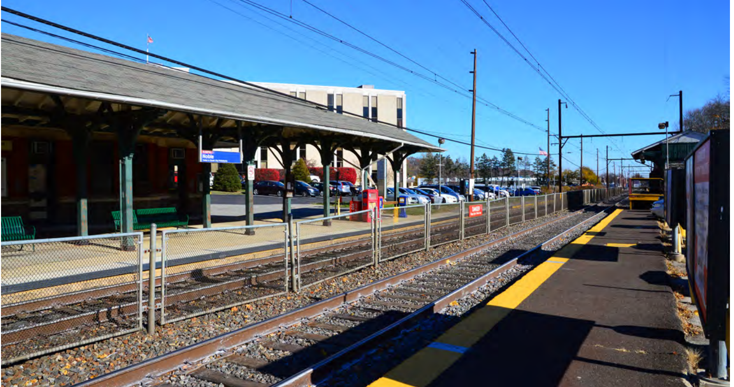
Looking east at Noble Station platform from the outbound track
