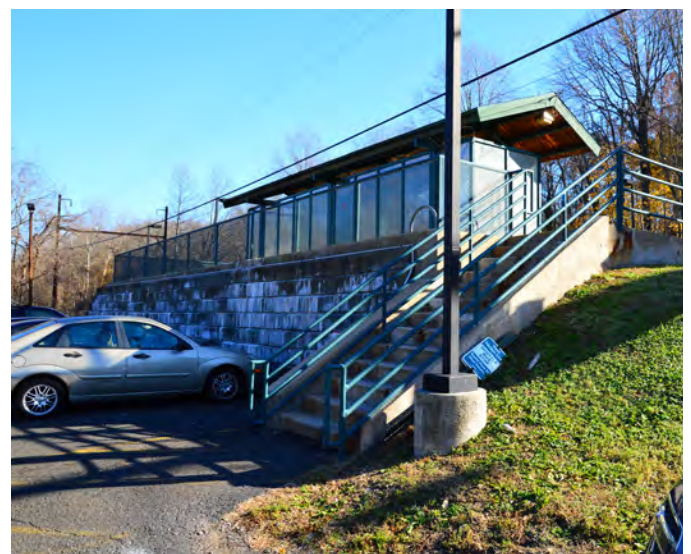
Meadowbrook Station platform, shelter, and parking area
