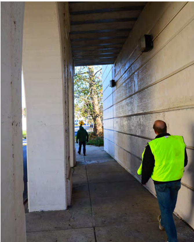
Sidewalk under rail bridge at North Hills Station
