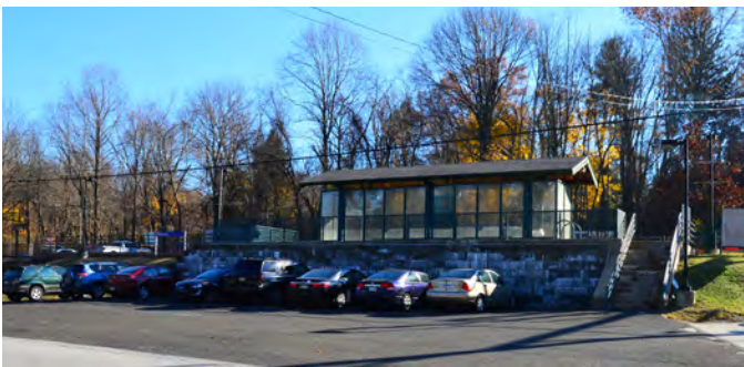
Meadowbrook Station platform, parking lot, and inbound track shelter
