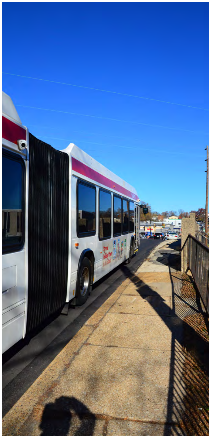
Sidewalk on bridge over Noble Station
