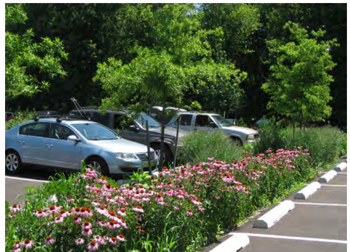
Example of a parking lot rain garden
