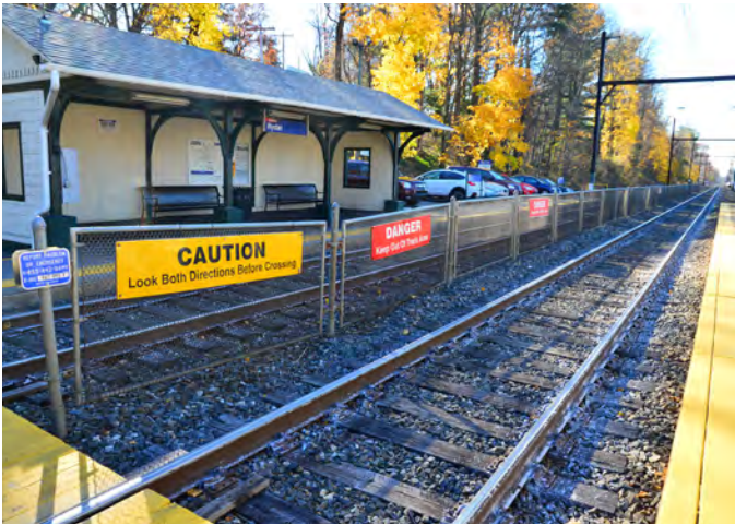
Platform, rails, and rail crossing at Rydal Stations
