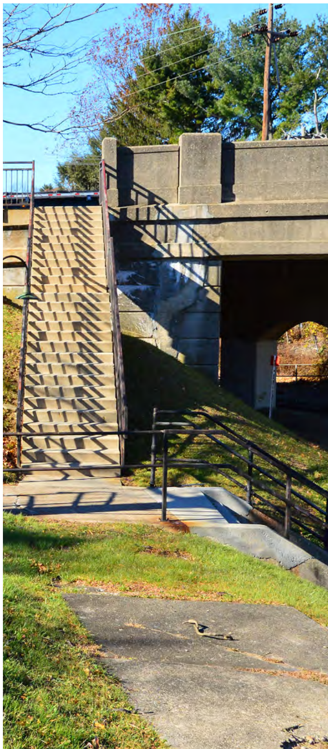
Stairs to Old York Road at Noble Station
