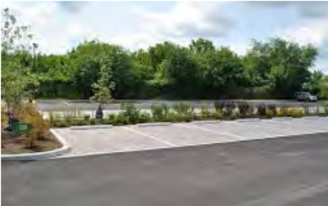
Example of a parking lot with permeable pavers and pervious pavement
